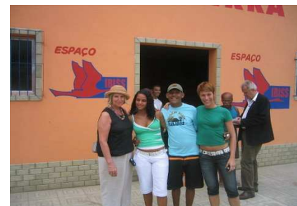
The almost completed Community Center
